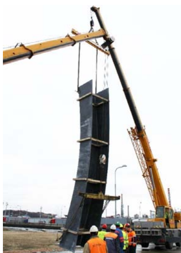
Fig. 14 Rotation of footbridge I
