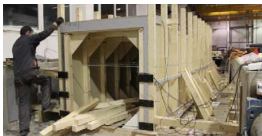
Fig. 12 Wooden formwork of footbridge I
