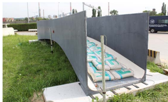
Fig. 19 Perform static loading test on footbridge II
