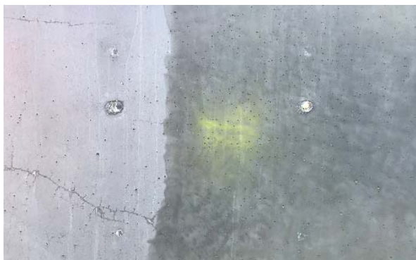
Fig. 22 Surface after brushing
