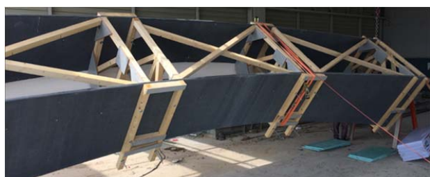
Fig. 18 Rotation of footbridge II
