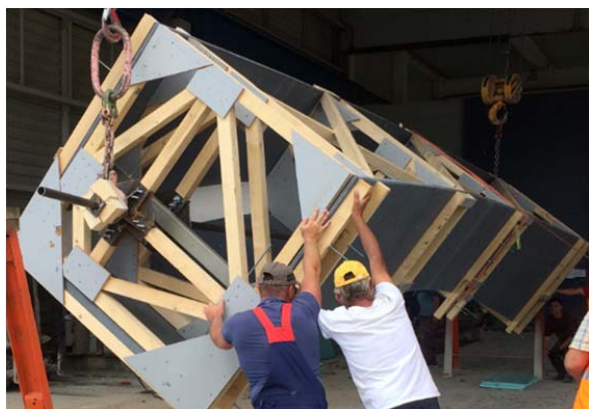
Fig. 17 Rotation of footbridge II
