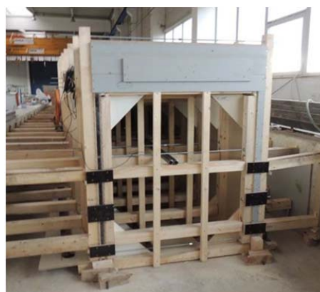
Fig. 16 Formwork of footbridge II
