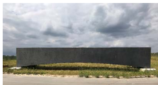
Fig. 25 Final visage of footbridge II
