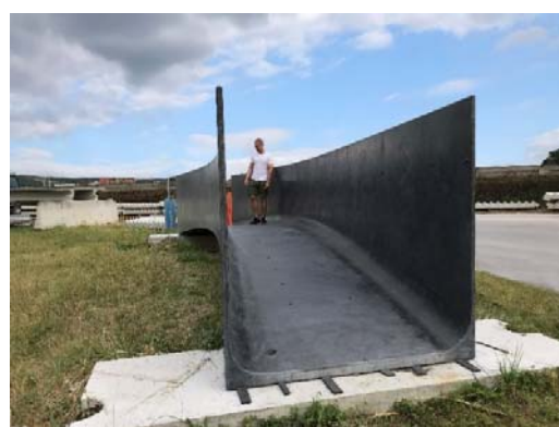
Fig. 26 Final visage of footbridge II
