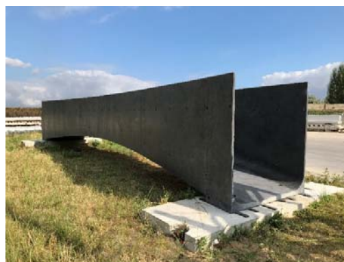
Fig. 24 Final visage of footbridge II
