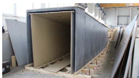
Fig. 13 Removing of wooden formwork
