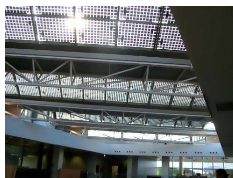
Fig. 7 Isofóton, Spain. Detail of the monocrystalline cell modules [10]
