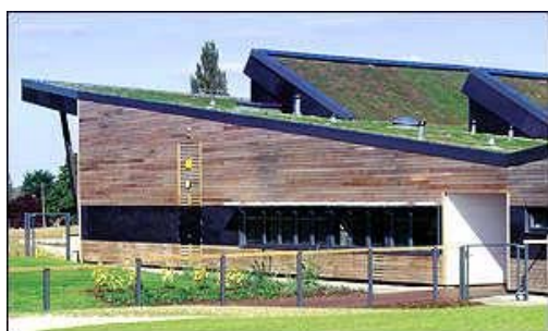
Fig. 3 Covered with green roof and accesses of natural light [7]
