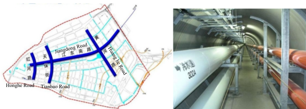
Fig. 4 Underground comprehensive pipe corridor of Hexi New Town
