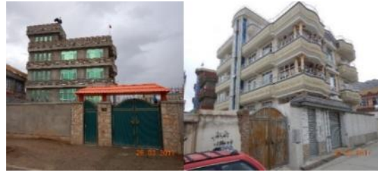
Fig. 9 (c) Private investments (four- and five-story) after ISU at Site B
