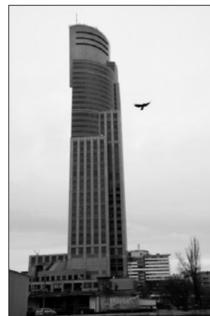
Fig. 3 Warsaw Trade Tower
