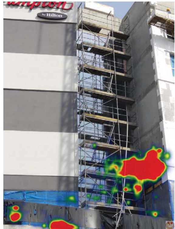
Fig. 3 Heat map scaffolding L13
