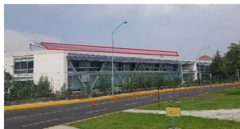
Fig. 3 Photography of the C3-UNAM Building rooftop PV System, University City. Image by Viridiana Ardura Perea
