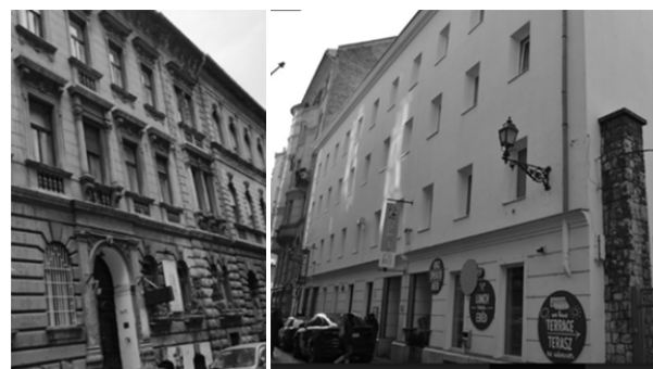
Fig. 4 Traditional building with original decoration, and a same age building with external insulation on a historical building,
