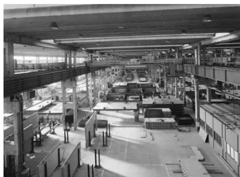
Fig. 2 Prefabricated sandwich panel factory in Hungary, 1974 [15]
