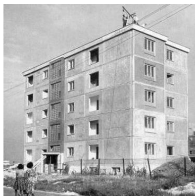
Fig. 1 First 'panel' building in Hungary [14]
