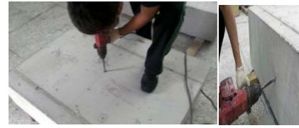
3. Concrete hole drilling
