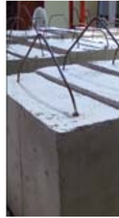
2. Construction of concrete specimen
