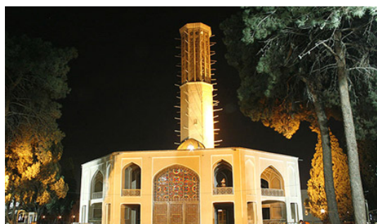
Fig. 2 Windward is one of the key elements of Iranian architecture. This is the Dolat Abad wind ward and the highest one in the world [11]
