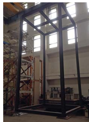
Fig. 2 The steel frame
