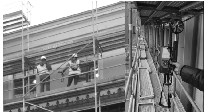
Fig. 3 The measurements on the scaffolding
