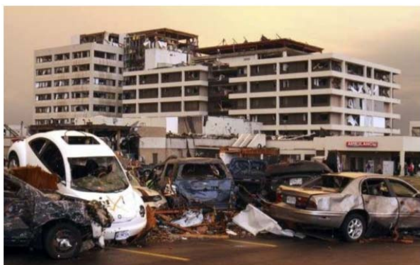
Fig. 6 Impact of Joplin Tornado on SJRMC [14]
