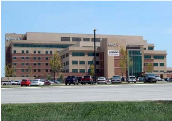
Fig. 9 New Hospital after the Tornado [25]
