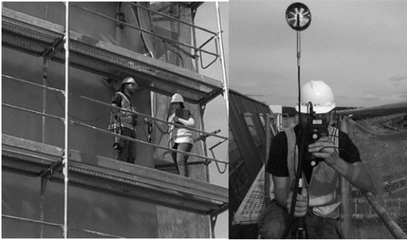
Fig. 1 The measurements on the scaffolding
