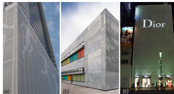
Fig. 1 Example of installing a perforated panel with pictures (a) Chicago Arkadia Apartment (b) Nordstjerneskolene state school (c) Tokyo Dior store
