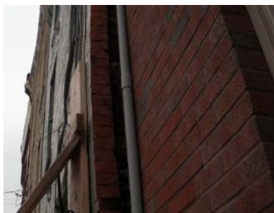
Fig. 2 New plumb wall next to old bulged brick
