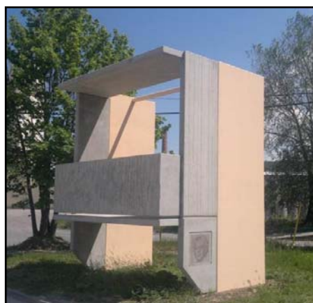
Fig. 4 Real construction of a self-supporting loggia
