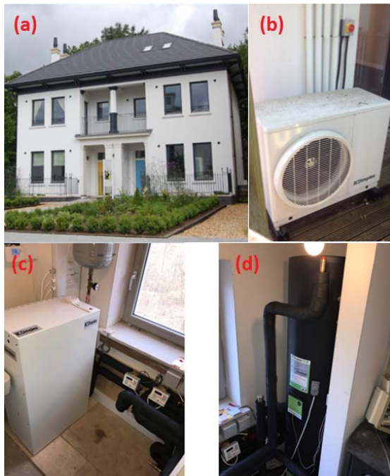
Fig. 2 (a) Building Research Establishment (BRE) Natural House, (b) Glen Dimplex heat pump, (c) Glen Dimplex Quantum Boiler, (d) Hot water storage tank
