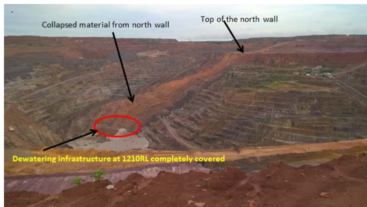
Fig. 6 KOV pit North wall after the Collapse in January 2016
