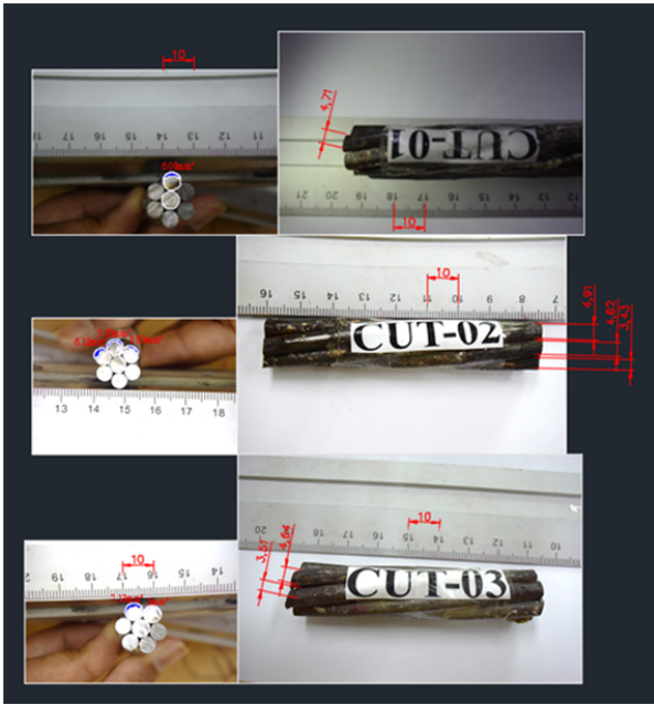
Fig. 3 Evaluation of corroded section
