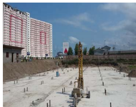
Fig. 4 Project site after the implementation of micropile
