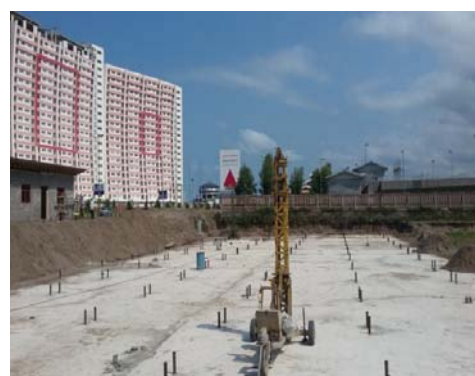
Fig. 4 Project site after the implementation of micropile
