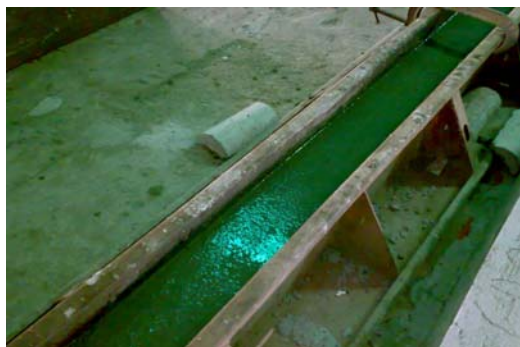
Fig. 2 Model steel reinforced bridge girder, after placing of concrete
