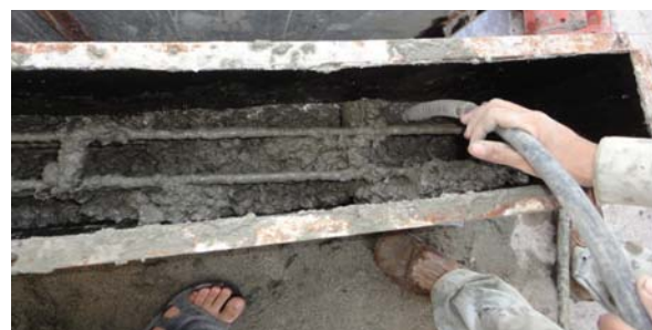
Fig. 4 Compaction of concrete in moulds with vibrator
