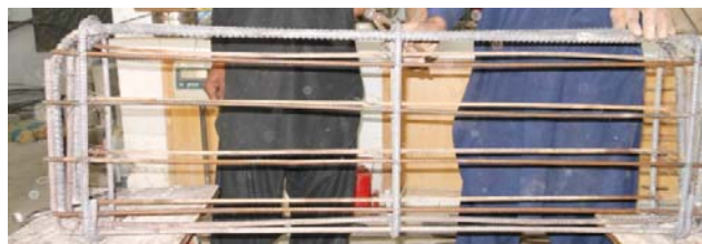
Fig. 3 Steel skeletons for beam specimens
