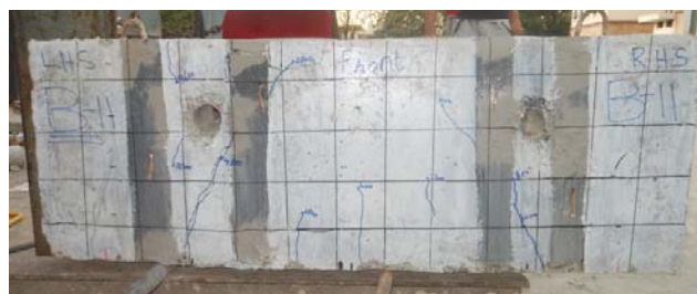
Fig. 10 Crack pattern of beams with opening above NA
