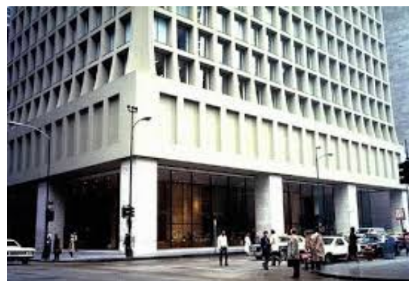
Fig. 2 Continuous deep beams supported on concrete columns
