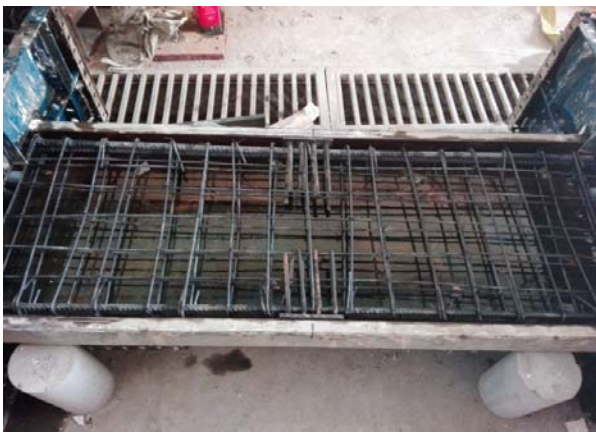
Fig. 4 Detail of reinforcement in deep beam
