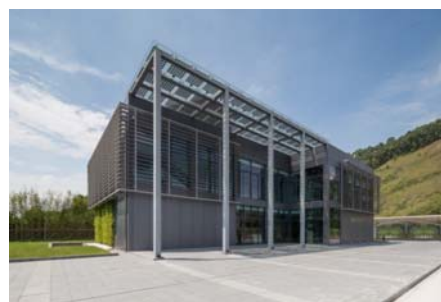
Fig. 3 The entrance of the test office building (north view)
