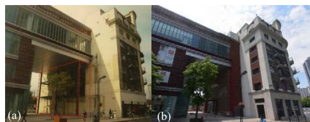
Fig. 6 (a) Photo of the south façade of Hongkou Building before renovation taken on 2012, (b) after renovation taken on 2016
