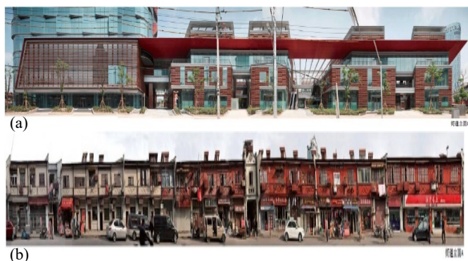
Fig. 3 (a) South façade of commercial annex, (b) the façade facing across the road
