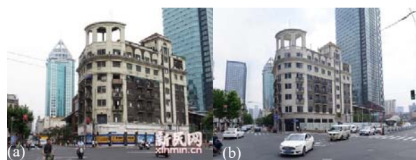
Fig. 5 (a) Photo of Hongkou Building from the intersection of North Sichuan Road and Haining Road before renovation taken on 2012, (b) after renovation taken on 2016
