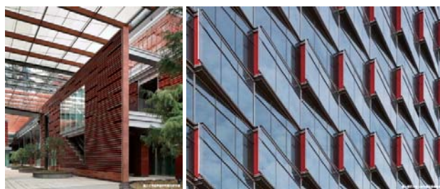
Fig. 10 (a) Clay pipe surface, (b) red surface of vents in high-rise office building
