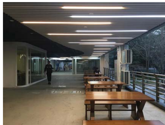
Fig. 14 Ceiling with linear lights
