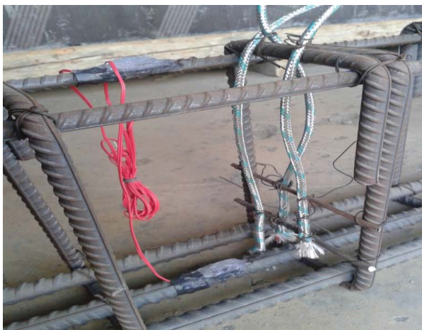
Fig. 2 Location of thermocouples at beams midspan
