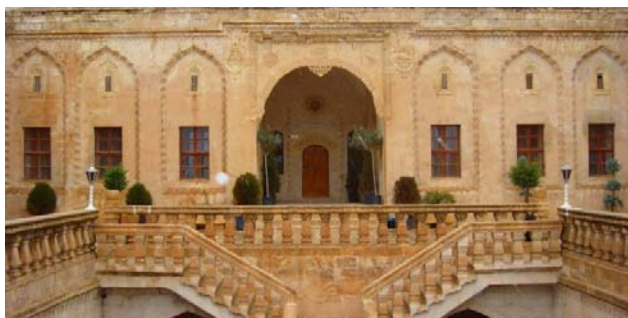
Fig. 8 Facade of Mardin PTT House
