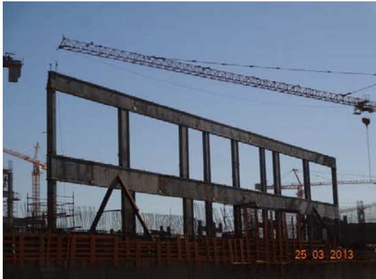
Fig. 4 (b) Installation of steel beams and columns (ground floor view)
