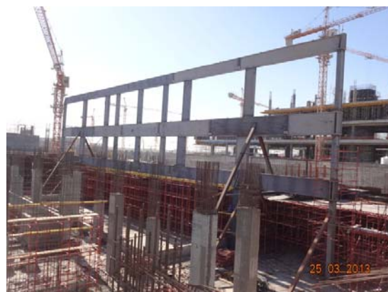
Fig. 4 (a) Installation of steel beams and columns (basement view)
