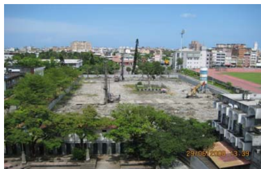
Fig. 1 Excavation construction site
