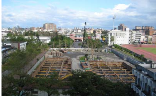
Fig. 2 Excavation construction support
