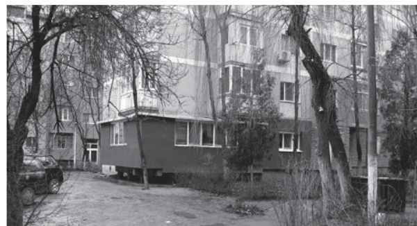
Fig. 17 Private ground floor extension
