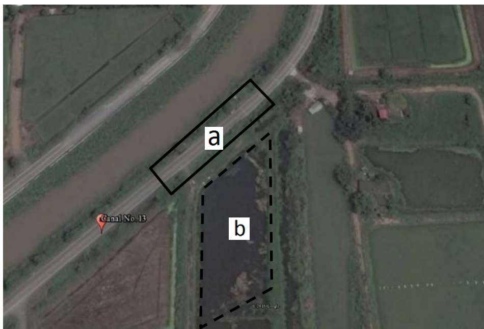
Fig. 2 a. The collapsed areas b. Shrimp ponds
