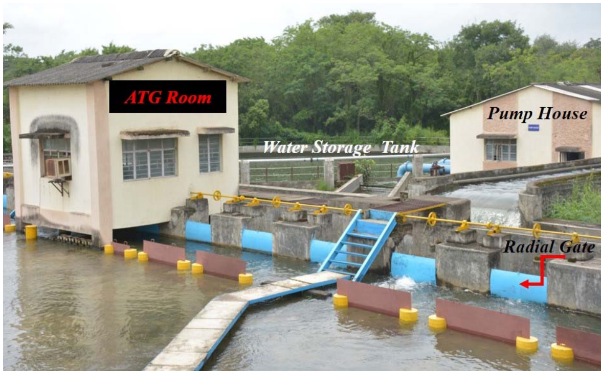
Fig. 4 Automatic tide generation system
