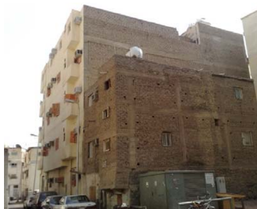
Fig. 3 Photo of the studied building in Madinah
