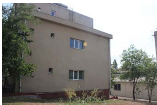
Fig. 6 (a) The appearance of the northern façade of the sample building
