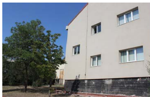
Fig. 9 (a) The bare façade
