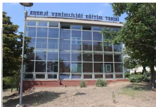
Fig. 6 (b) The appearance of the southern façade of the sample building
