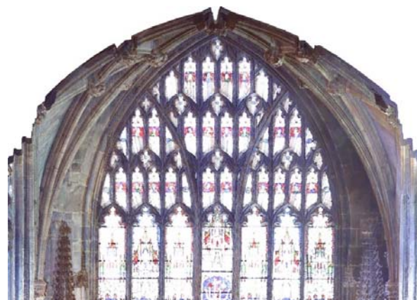
Fig. 7 Orthophoto short section created using a point cloud to demonstrate the rib curvature in the chancel of St Mary's, Nantwich
