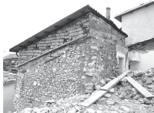
Fig. 3 Typical residential building
