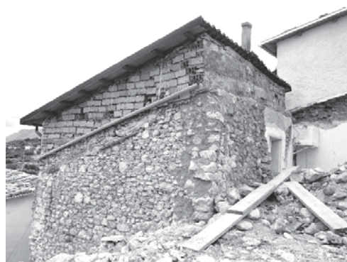
Fig. 3 Typical residential building
