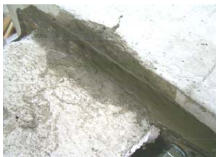
Fig. 3 Column-beam interface detail
