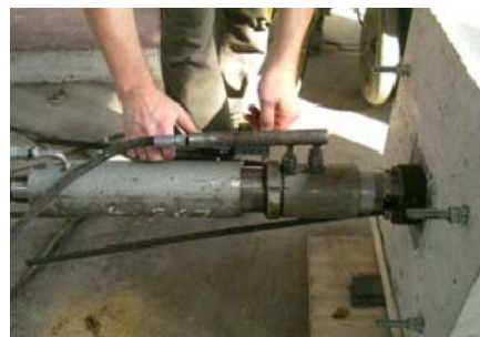
Fig. 4 Pre-stressing of the strands
