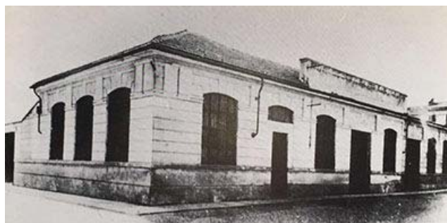
Fig. 16 Historical image showing part of the LANCIA buildings in 1911
