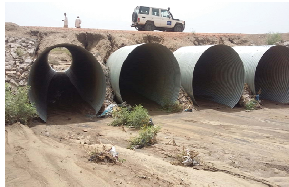
Fig. 8 Sediment deposition and vegetation in the apron area
