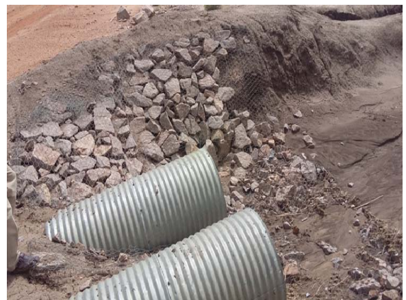
Fig. 9 The gabion mesh used for lining of wing walls
