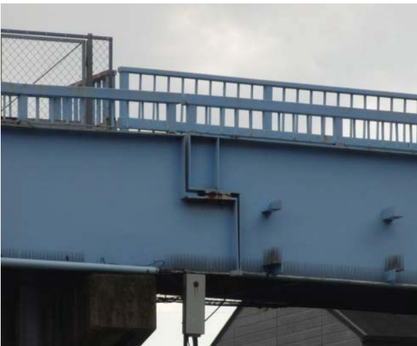
Fig. 2 Hinge connection at middle bridge pier
