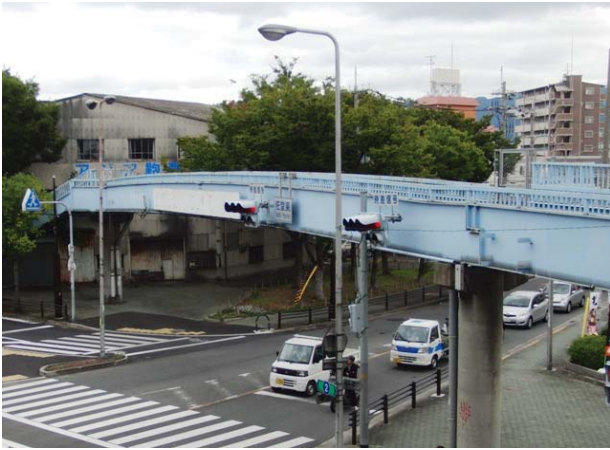
Fig. 1 Footbridge being tested
