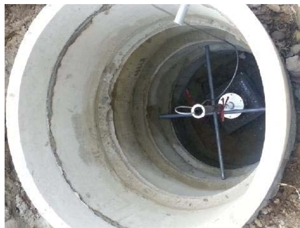
Fig. 2 A seismometer was mounted on the concrete foundation with a depth of 2 meters in the second stage
