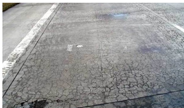
Fig. 1 Damage of top layer of the concrete road with RCA due to ASR
