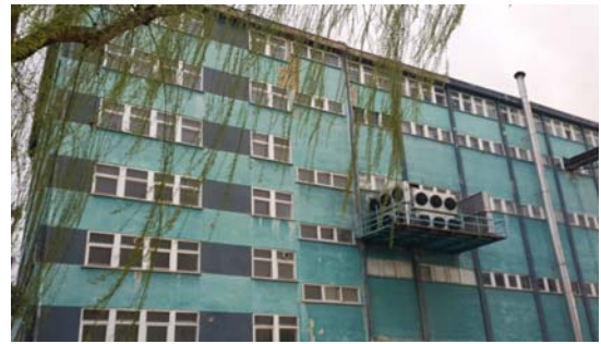
Fig. 9 Weak framed typical official building in Turkey
