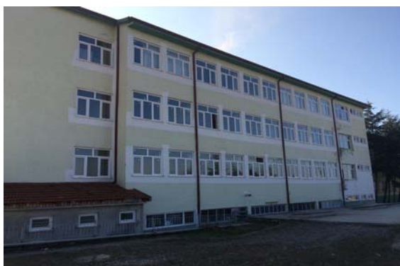
Fig. 3 Weak framed typical school building in Turkey
