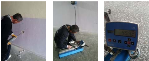
Fig. 8 Anchorage pull out test
