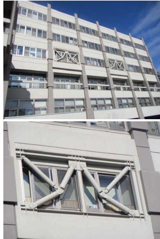
Fig. 1 Earthquake-Resistant Dampers for Building
