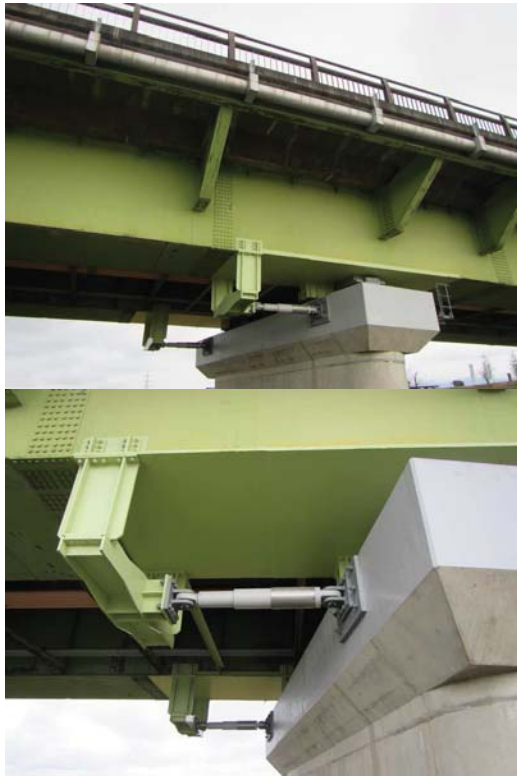
Fig. 2 Earthquake-Resistant Dampers for Bridge
