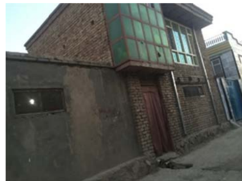
Fig. 12 Sample of masonry building
